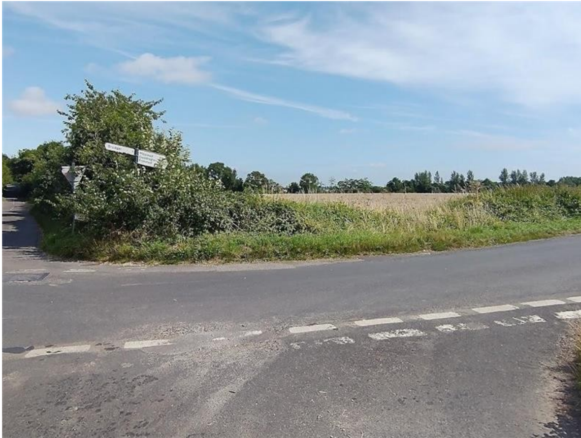
The site of the proposed M2 Junction 5A shown looking from Hawks Hill Lane at the junction with Bexon Lane and Ruins Barn Road.
